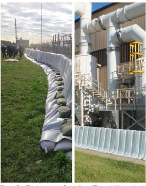
Figure 8. The temporary "muscle wall" erected to protect the PVSC treatment plan in July of 2013 would be replaced with a permanent flood wall as part of the PVSC's Flood Mitigation Plan. (Source: "Recovering from Superstorm Sandy," PVSC, January, 201
