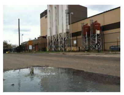
Figure 9. Passaic Valley Sewerage Commission Plant near Newark Bay was impacted by Sandy. This Star Ledger file photo shows raw sewerage bubbling up from ground.
